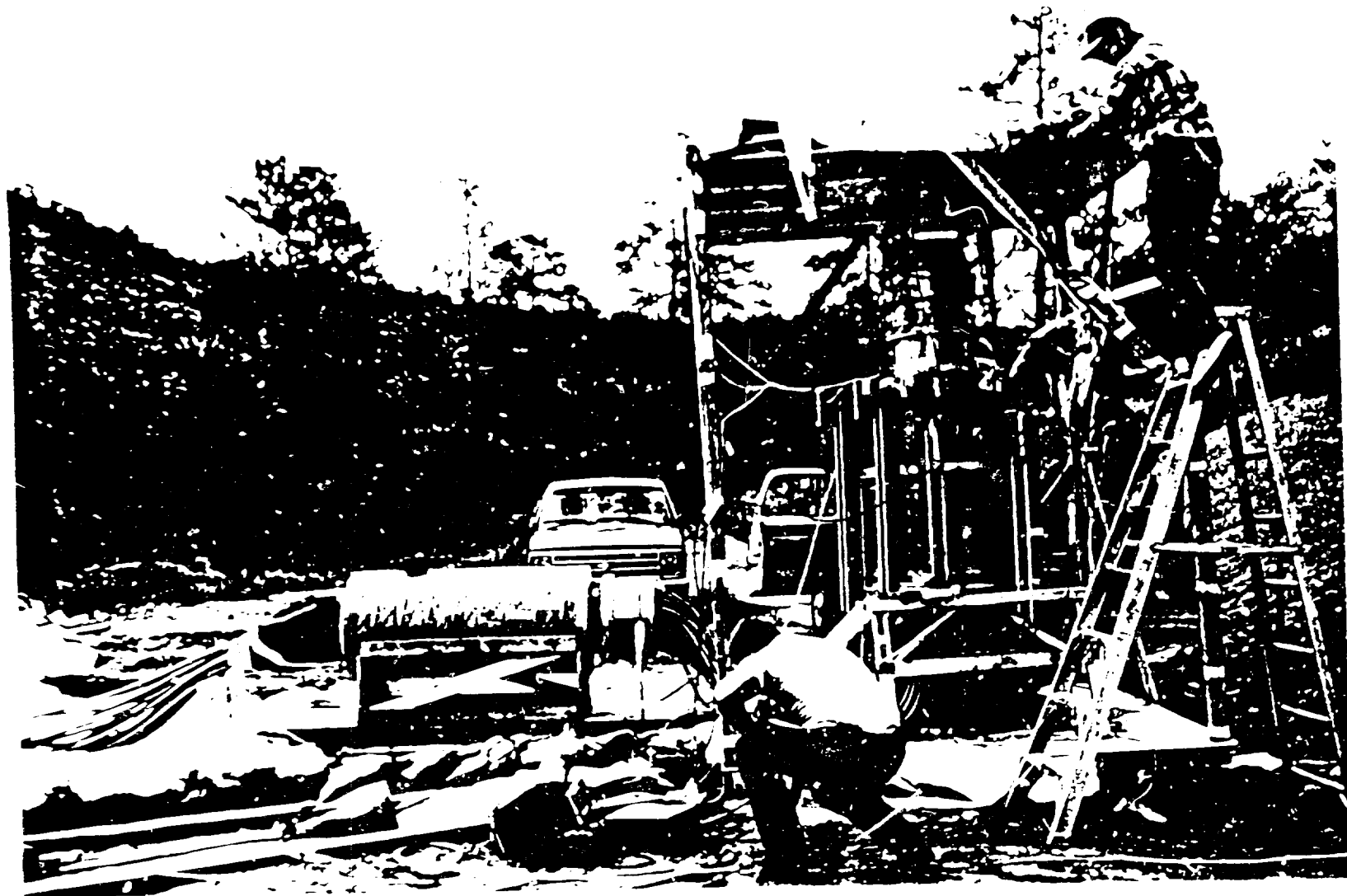
Fig. 1. The Laguna system being constructed at Firing Point 88, Los Alamos National Laboratory.
